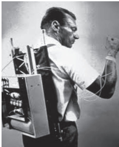
The first insulin pump (source: www.timestoast.com )
